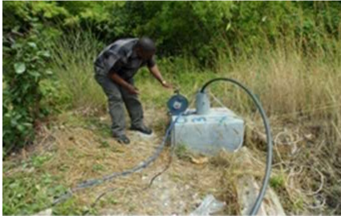
Figure5: Pumping test at borehole MJ7
